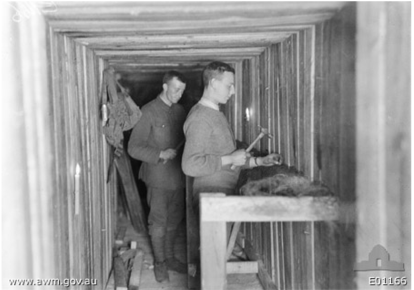
Nieuport-Bains, 13 November 1917 - Two unidentified members of the 2nd Australian Tunnelling Company fitting up bunks in the tunnels under the dunes near the Belgian coast. The unit was at the time attached to British troops operating in this sector.
