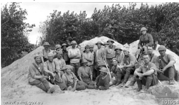
THE 2ND TUNNELLING COMPANY IN THE AFFAIR AT NIEUPOORT
