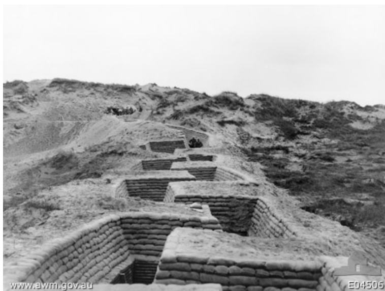
A sandbagged trench leading to the entrance of a tunnel (background, left). During June and July 1917 the 2nd Australian Tunnelling Company, attached to the 1st British Division, were engaged in constructing the defensive works in the Nieuport area. Note a group of unidentified soldiers standing outside the entrance to the tunnel.
