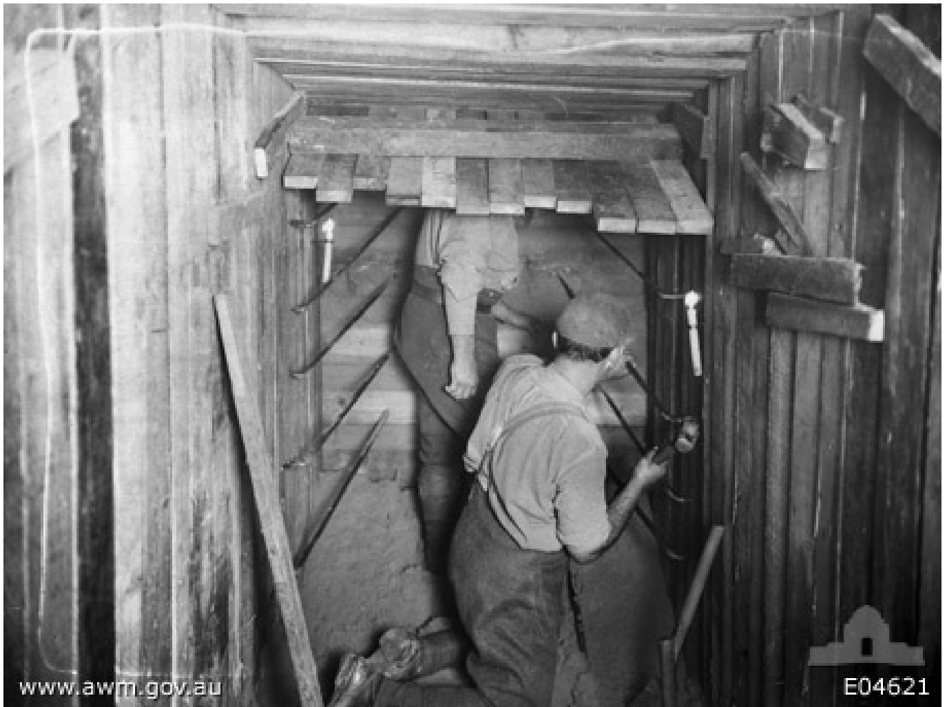
November 1917 - Two unidentified members of the 2nd Australian Tunnelling Company working by candlelight on a tunnel. A few months earlier the company, attached to the 1st British Division defending the area, was engaged in constructing defensive works in the Nieuport-Bains sector.
